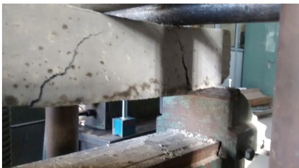
Fig.No. 2 Loading & failure of beam
