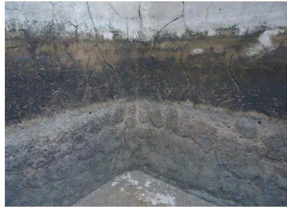
Plate I: Cracked walls of concrete fish
